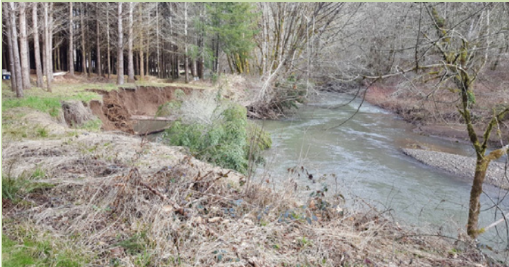
High flows during storm events caused streambank erosion along Greasy Creek south of Philomath.
