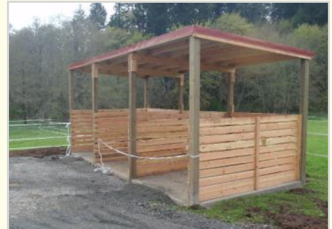
Manure Composting Facility
