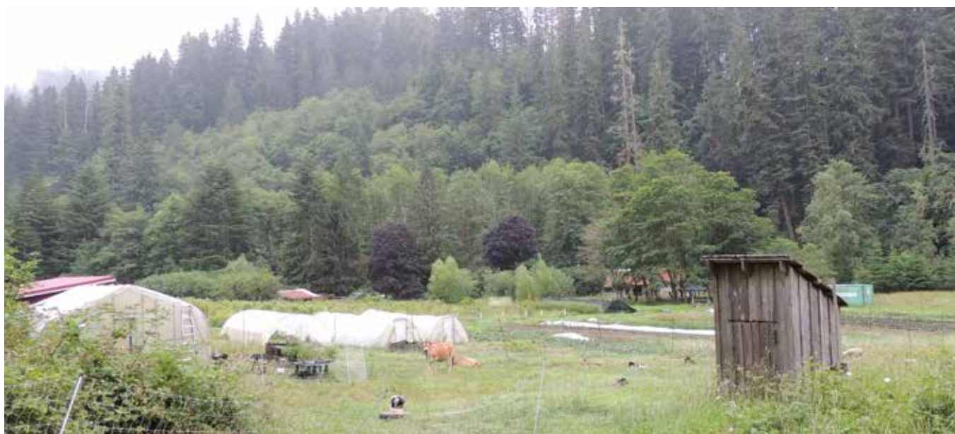
The wellhouse, at right, protects the well, pump, and water treatment equipment. 14
