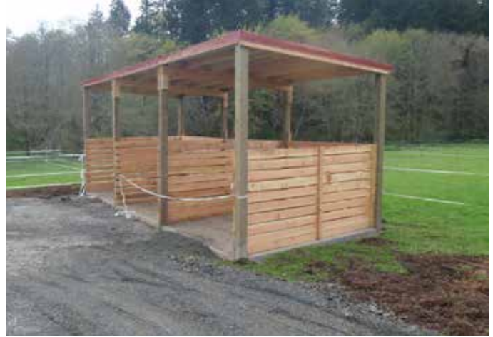
A three bin compost facility prevents manure runoff contamination to the nearby stream. 25
