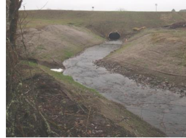
Newly constructed stream bed and fish-friendly culvert
