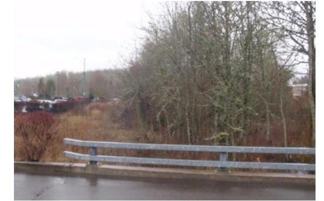
Intact streambanks help filter runoff from the parking lot.
