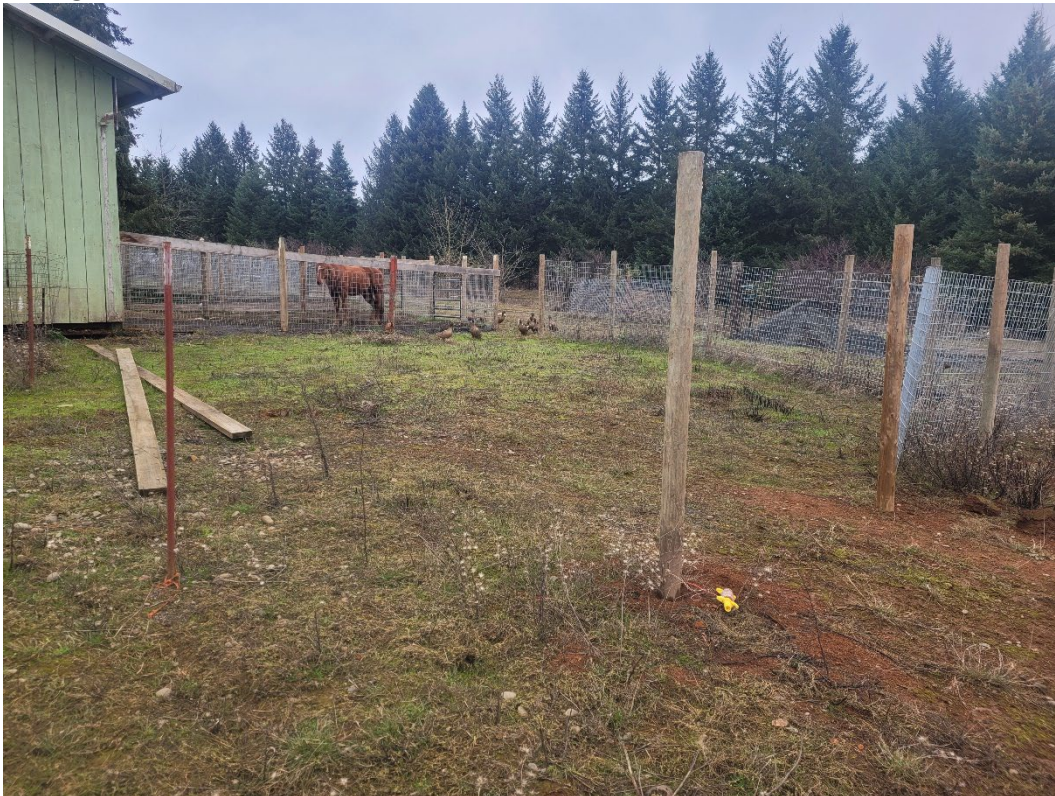
New gutters with French drains will direct clean water from the roof away from the area.
