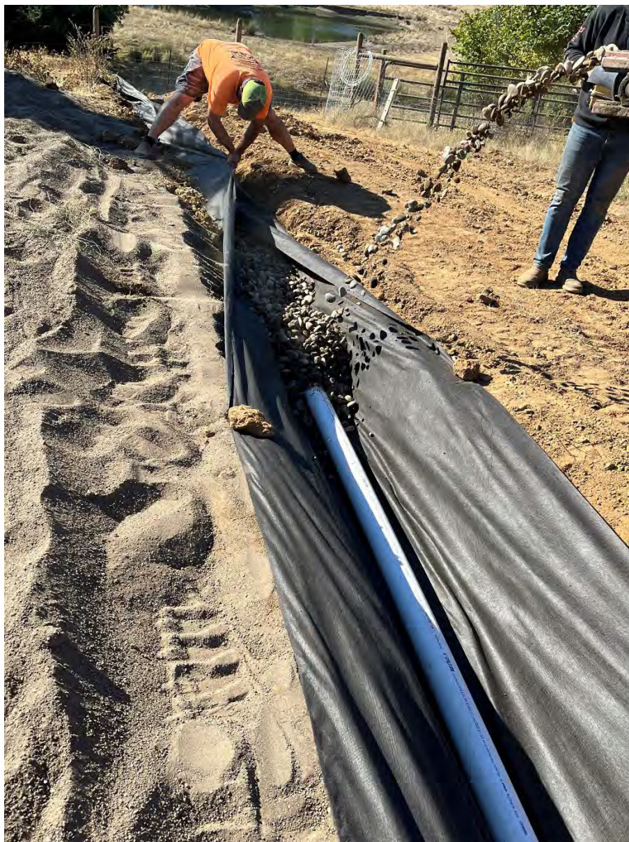
French drain installation-Jumping Giraffe Water Management project.
