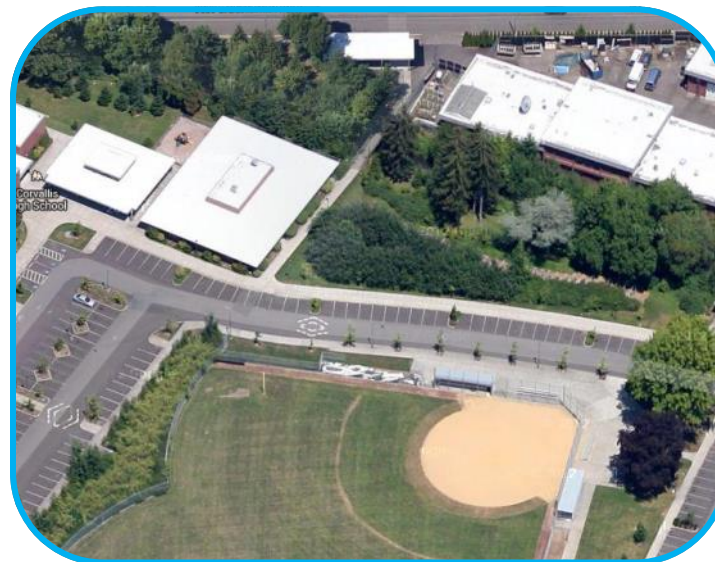
This aerial image from Google Maps shows the parking lot, bioswale, and creek on the CHS campus.
