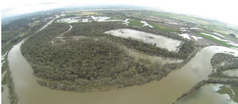
Photo 3: Aerial Flooding Photos- Bowers Rock State Park and Greenbelt Land Trust Little Willamette property during January 2012 flood event (Photo Credit: Calapooia Watershed Council).
